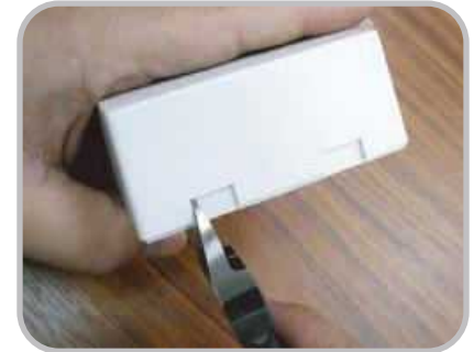
3. Use the cutter to cut one side of cable outlet
